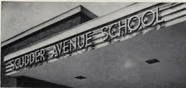
L-5: Bright satin finished sheet bronze letters to contrast with a stainless steel fascia.
